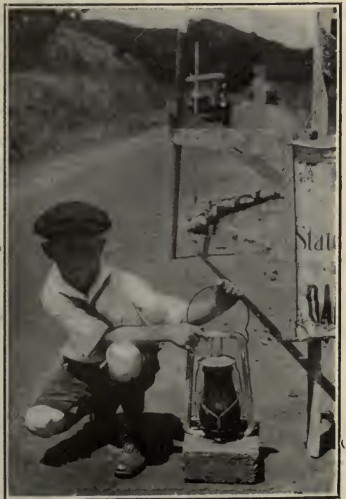
THIS LANTERN STAYS UPRIGHT—AND IS INCONVENIENT TO STEAL
